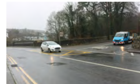
Desire Line 3: Difficult to cross station road.
