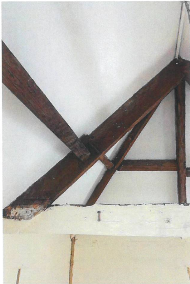
Exposed roof timbers in C01.
