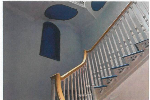
Niche to stairs between 1st and 2nd floor.
