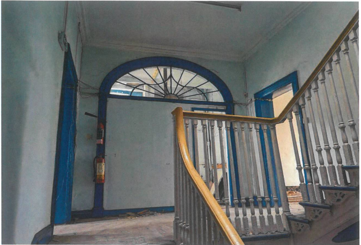
Stairwell S02 looking east.
