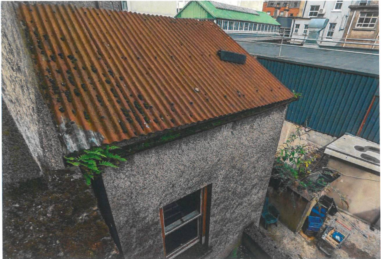
Roof of two storey addition at rear.
