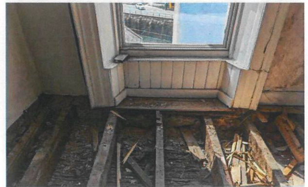
Window reveal and cill in T01.
