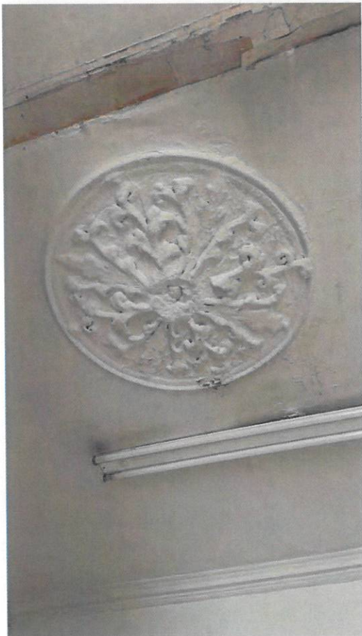
Ceiling rose and cornice detail.
