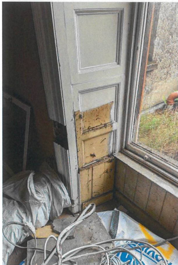
Window, reveal and architrave.
