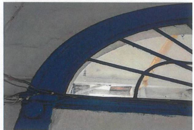
Detail of fanlight glazing.
