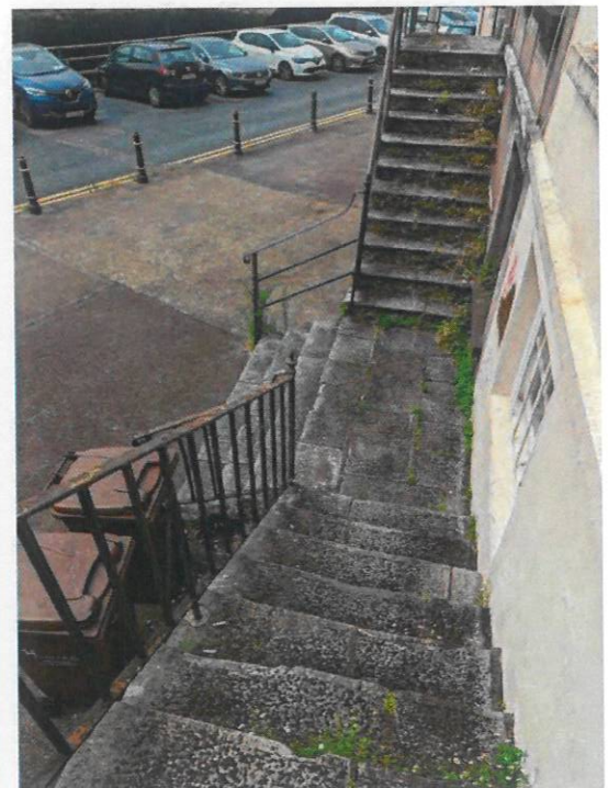
Steps and railings to south elevation.
