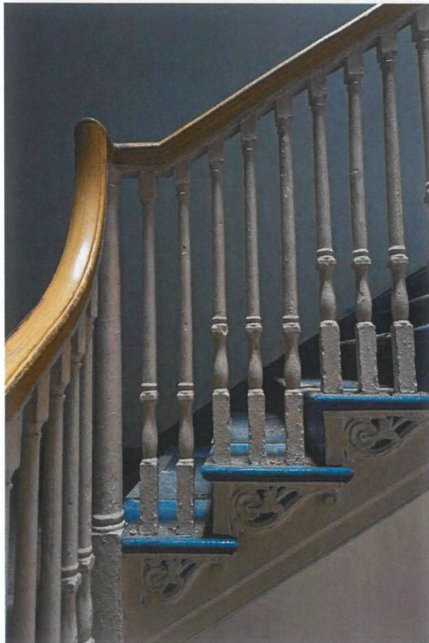
Detail of stairs.
