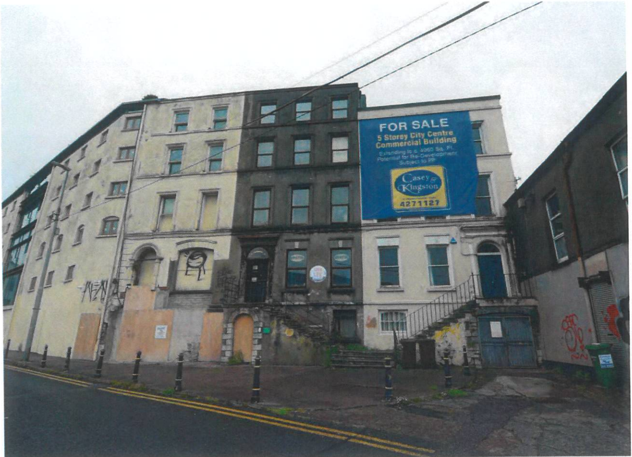
Front (south) elevation showing neighbouring properties.
