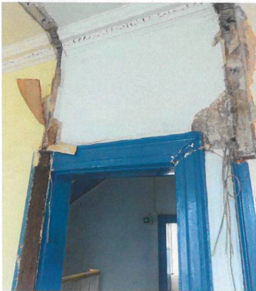
Door architrave and partition scars in S01.
