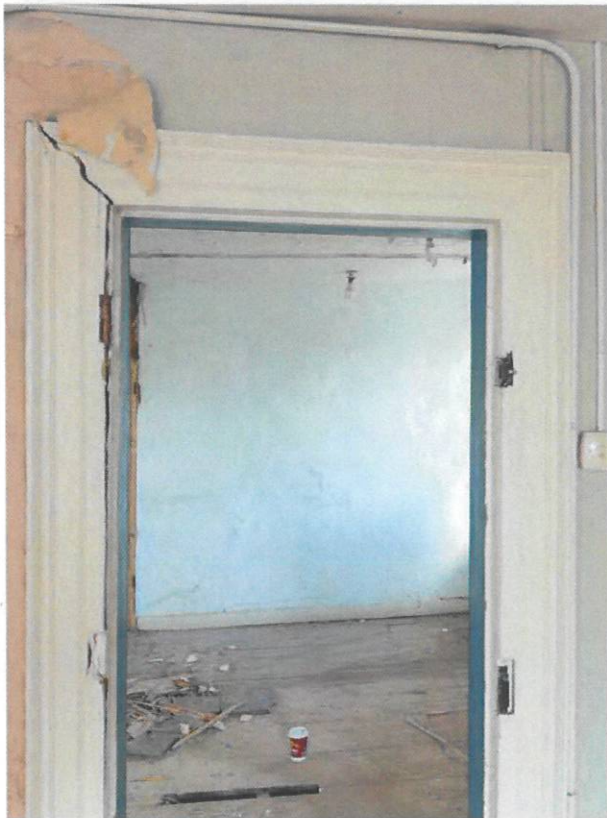
Detail of door architrave in T01.
