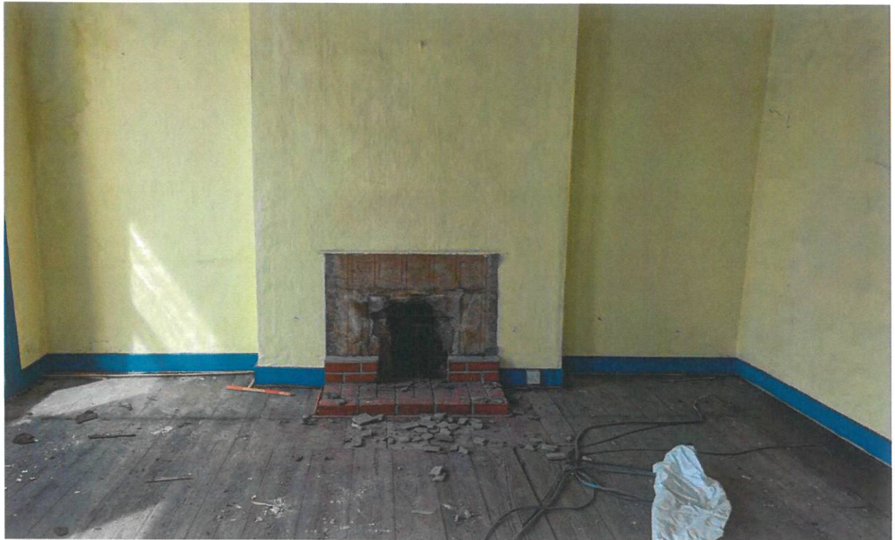
Room S01 looking west.
