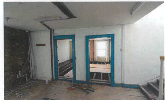
Room T02 showing twin doors to S01 at south.
