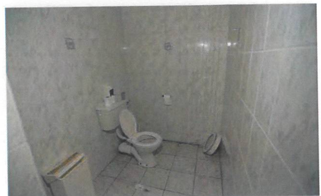
Room G05 looking north.
