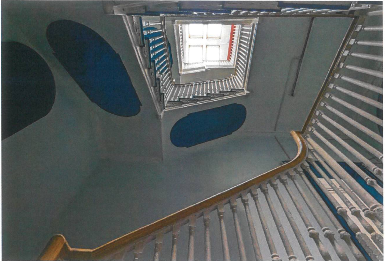
Stairwell looking up from F02.
