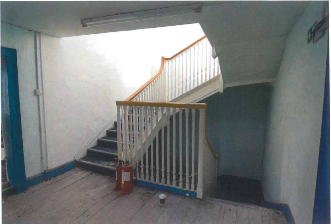
Room T02 looking towards stairs.
