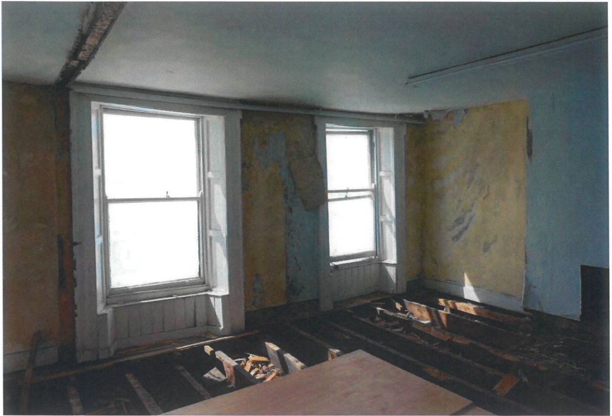
Room T01 looking southwest.
