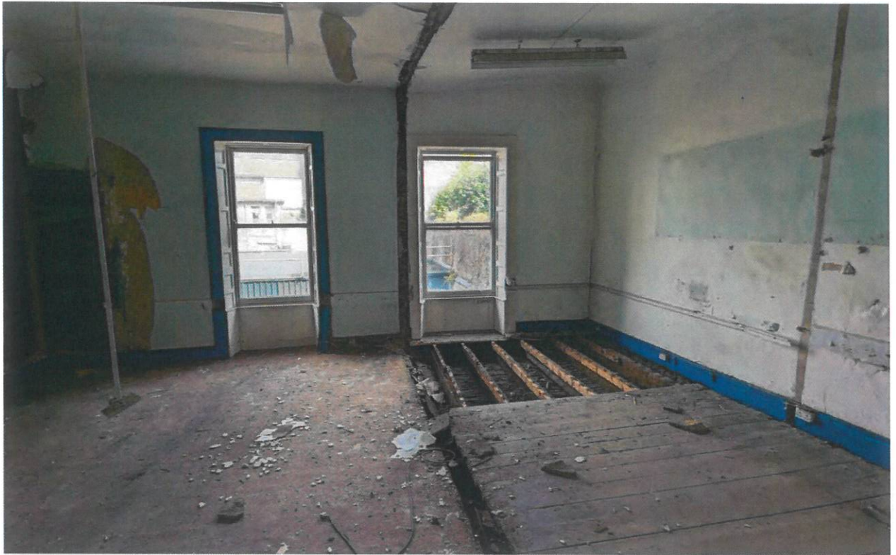
Room S04 looking north.
