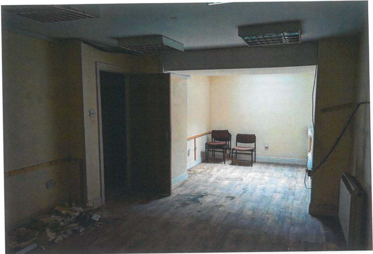
Room G04 looking north.
