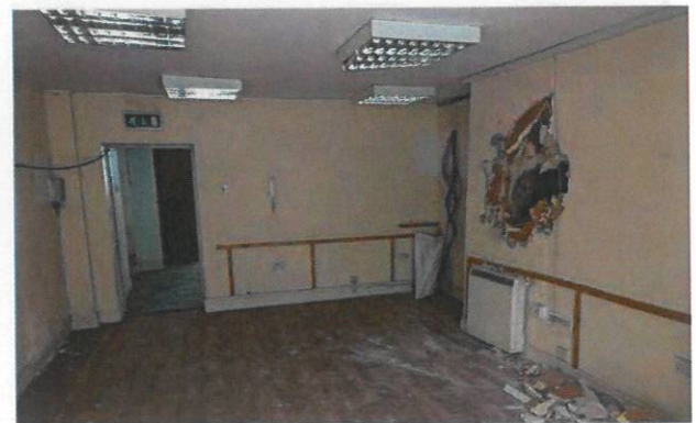
Room G04 looking south.
