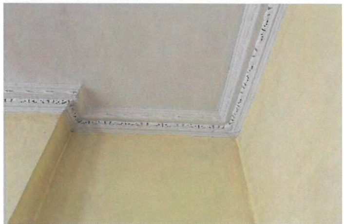
Plasterwork to room S01.
