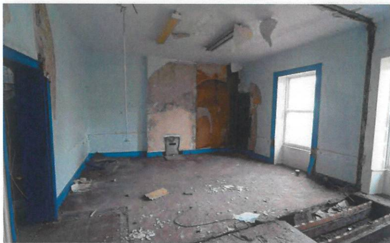
Room S04 looking northwest
