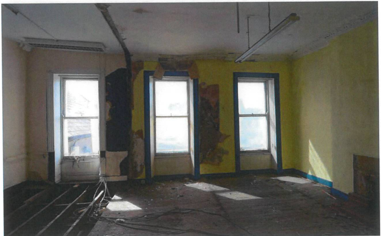
Room S01 looking south.
