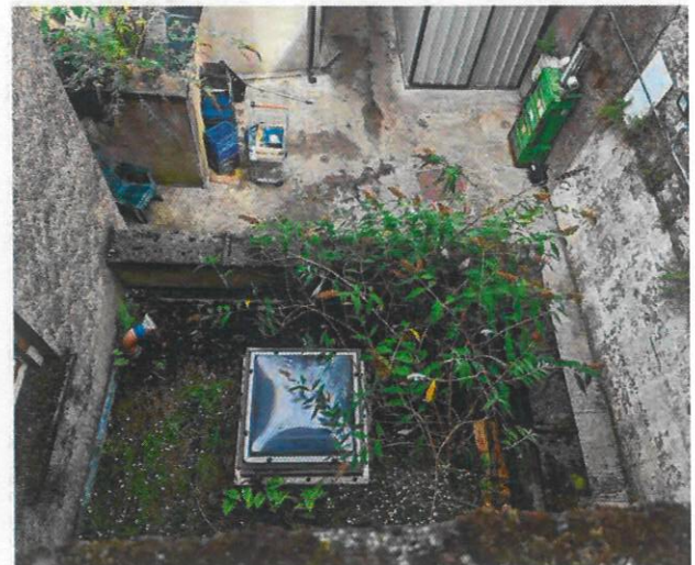
Roof of single storey flat roof addition at rear.
