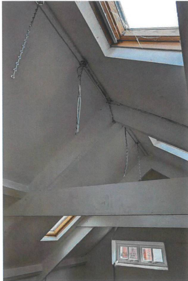
Exposed roof timbers in C03.
