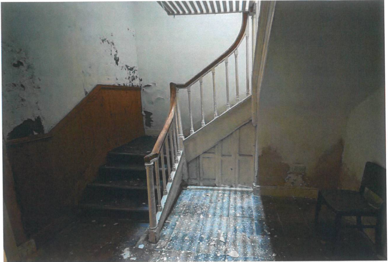
Stairwell G03 looking south west.
