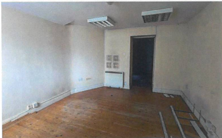
Room G02 looking north
