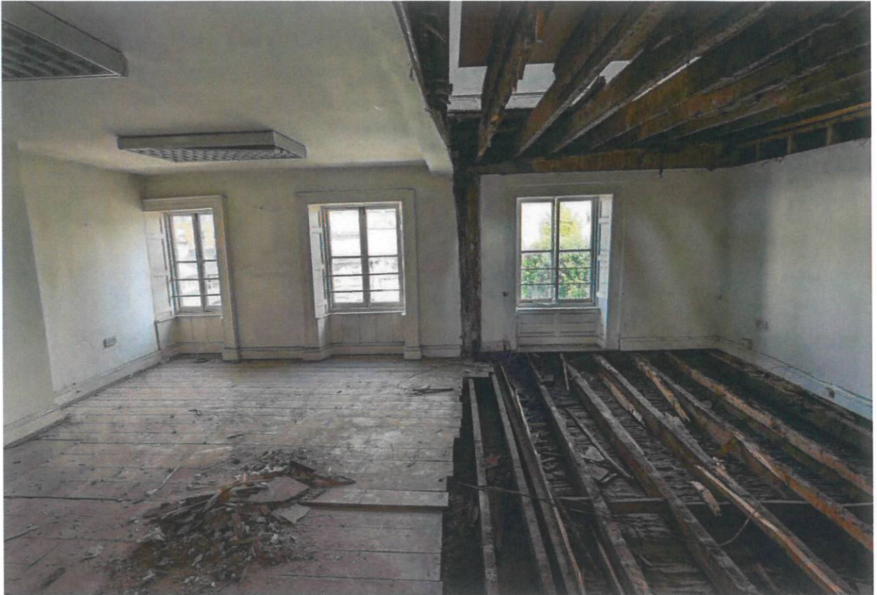
Room T03 looking north.
