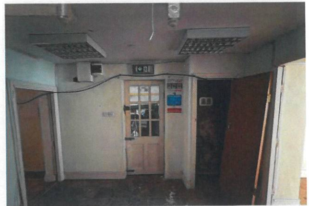
Room G03 looking east.
