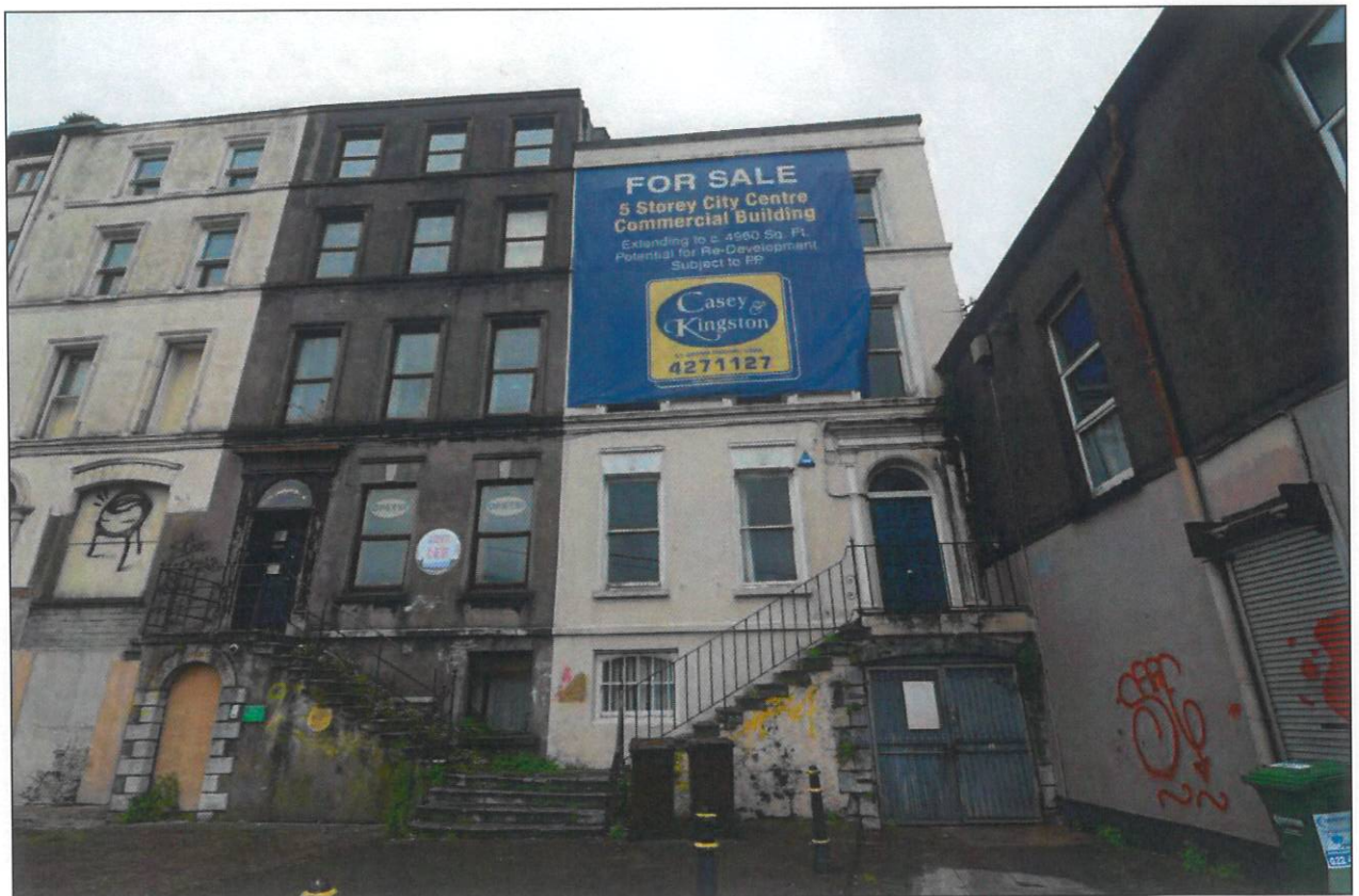
Figure 2: View 7 Fr Mathew Quay from the south (the building in question has the for sale sign).
