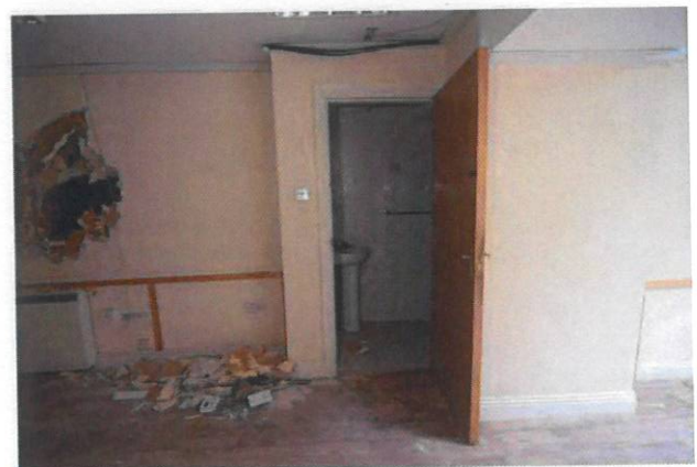
Room G04 looking west showing door to G05.
