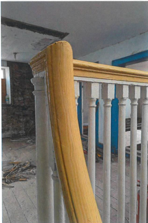
Detail of stair balustrade in T02.
