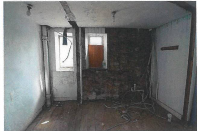
Room T02 looking east.
