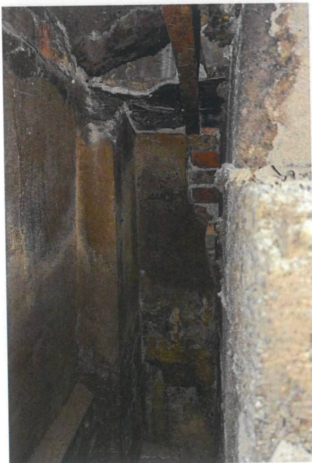
Interior of boarded up fireplace in G04.
