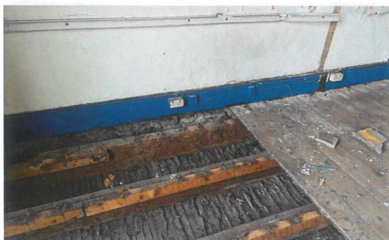
Partially Removed floor in S04.
