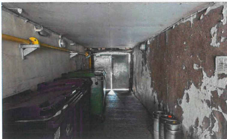
Passageway G02 looking south.
