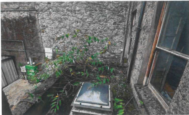
View from F04 over roof of G04 and windows to F03.
