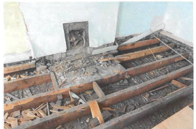
Fireplace and floor in T01.
