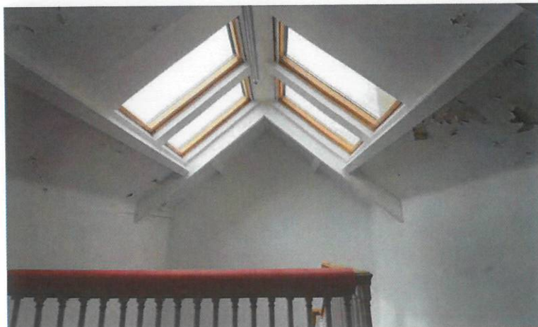
Rooflights in C02
