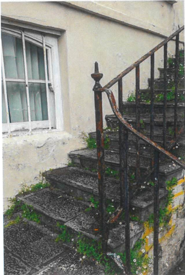
Detail of railing and limestone steps to front.
