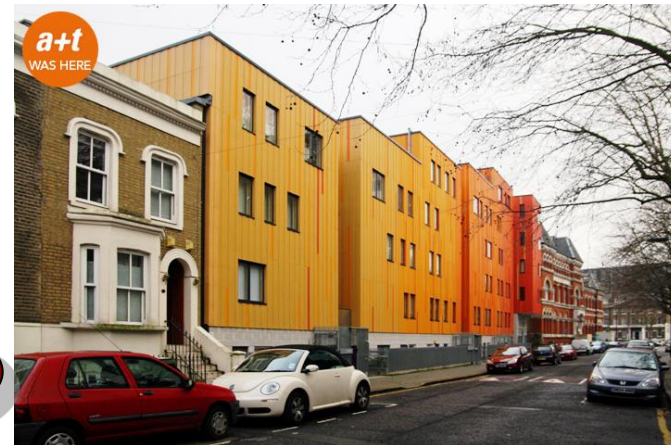
Innovative housing just built*
