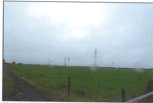
Plate 2-4 Kilbarry-Knockraha No. 2 110 kV Line crossing agricultural grassland (GAI)
