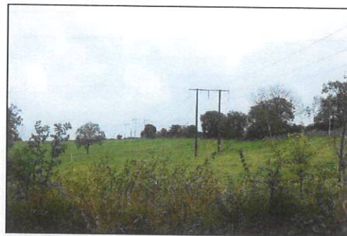
Plate 2-6 Kilbarry-Knockraha No. 2 110 kV Line crossing agricultural grassland (GAI)
