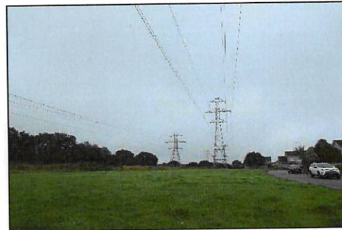
Plate 2- 14 Kilbarrý-Knockraha No. 2 110 kV Line crossing amenity grassland (GA2)
