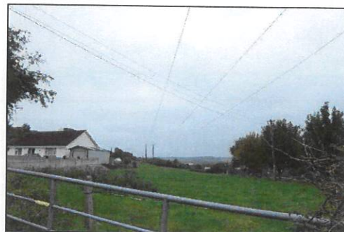
Plate 2-8 Kilbarry-Knockraha No. 2 110 kV Line crossing agricultural grassland (GAI)
