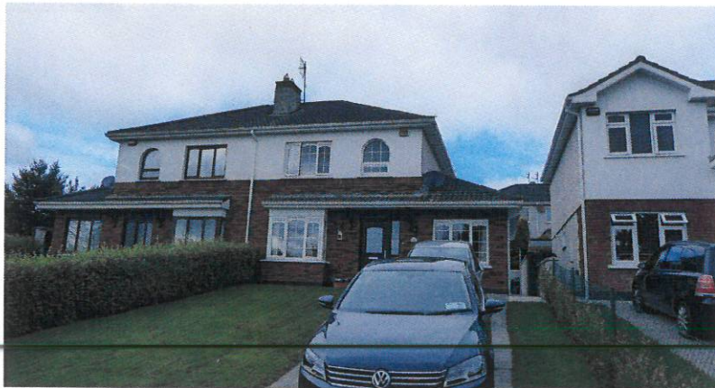
24 Oakfield Avenue, Glanmire, Cork, front of existing house
