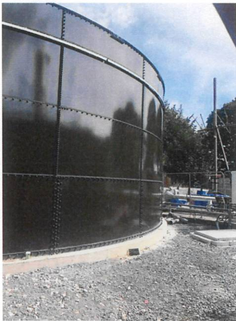
Plate 5 – Water tank as constructed facing south east
