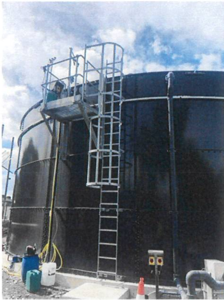
Plate 3 – Access ladder facing west
