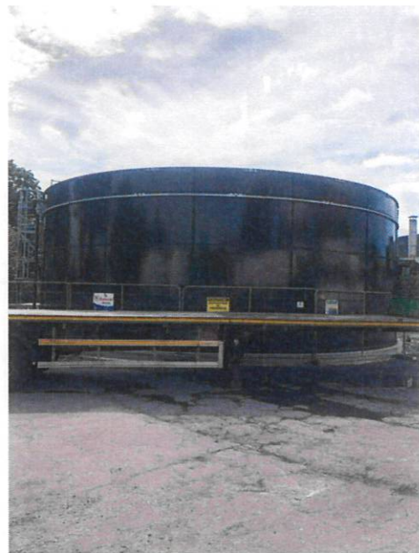
Plate 6 – Water tank as constructed facing south
