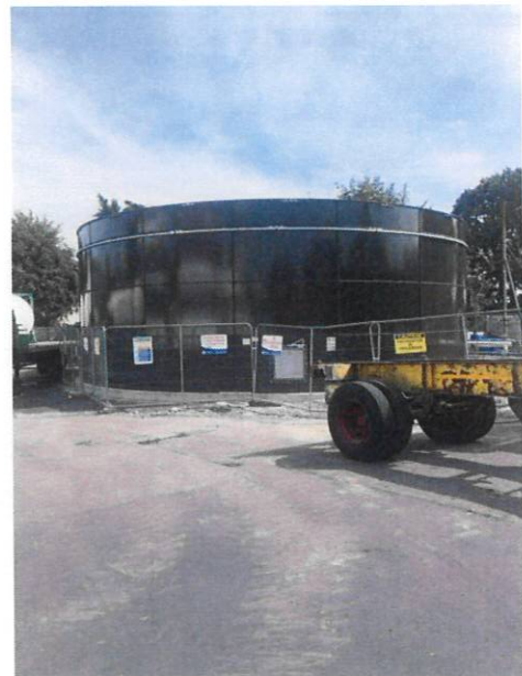
Plate 2 – Tank facing south east
