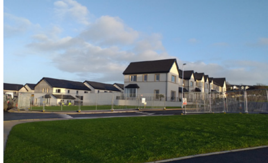
Housing development under way, Ballinglanna, Glanmire
