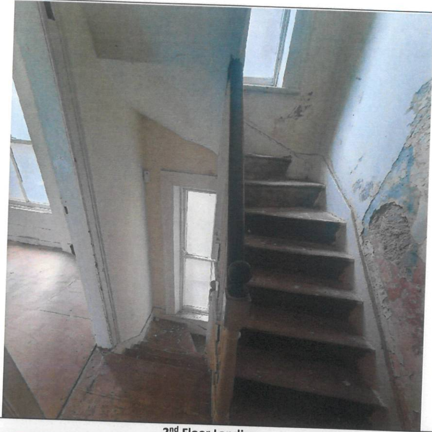
2 nd Floor Landing
