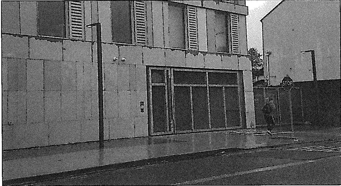
Plate 4. Side Entrance on Western Road
