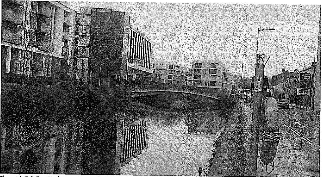
Figure 4: Existing Student Accommodation at Amnis House, Western Road, Cork.
