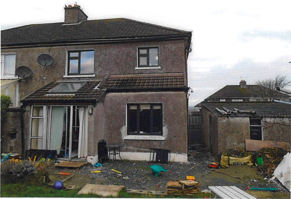
Image 2 – Rear Elevation 23 Earlwood Estate 11.01.2019
