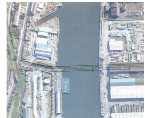
Water Street Bridge
