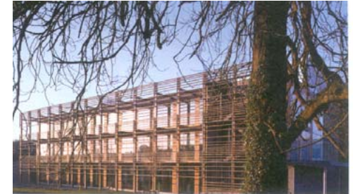
Passive Solar Design Aras An Chontae, Tullamore
