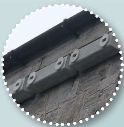
Double nest-cavity Schwegler Swift nest boxes installed at Mullingar Courthouse
