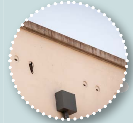
Swift investigating Swift brick nest boxes at Westport Town Hall
