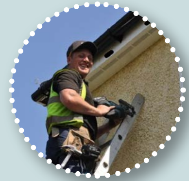
Swifts need an entrance hole to access an inner cavity which can be created in the fascia or soffit
