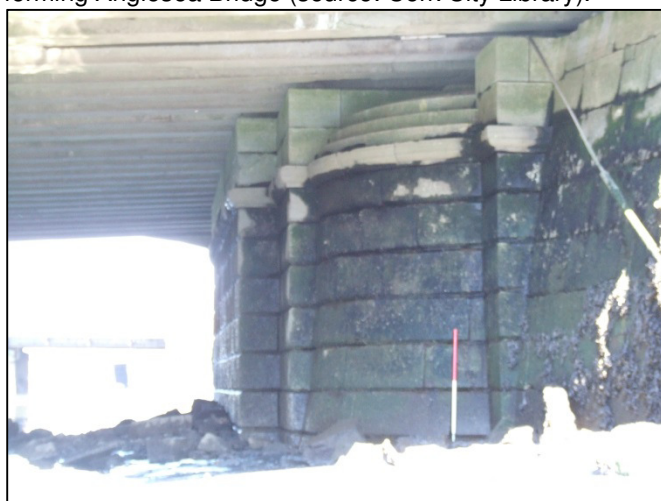
Plate 33: East-facing view remains of southern bridge abutment beneath the existing Parnell Bridge (1m scale).
