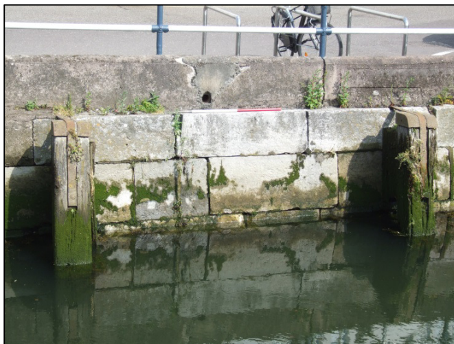
Plate 16: Example shot showing the top components of the timber fenders used along Father Matthew Quay/Morrison's Quay (1m scale).
