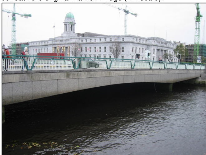
Plate 36: North-facing view upstream side of the modern Parnell Bridge built in 1971.
