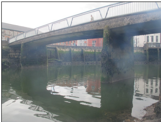
Plate 7: Southwest-facing view of the river channel at Trinity Footbridge.
