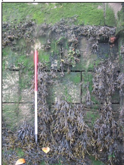
Plate 9: Detail shot of masonry used to construct Morrison's Quay (1m scale).
