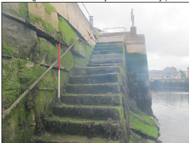
Plate 18: Example shot showing one of three identical sets of river-access steps located along Father Matthew Quay/Morrison's Quay (1m scale).
