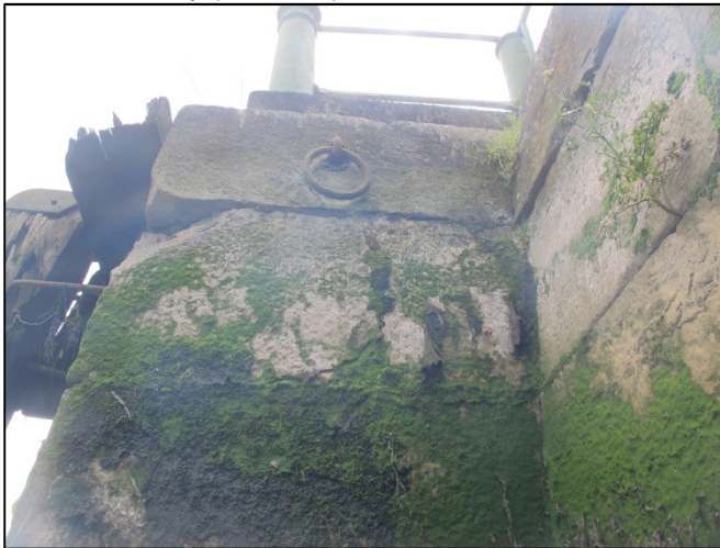
Plate 23: Example shot of smaller type of iron mooring hoop associated with the river-access steps along Father Matthew Quay/Morrison's Quay.
