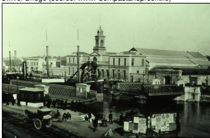
Plate 32: Twentieth-century photograph of the iron swivel-bridge that replaced (1882) the earlier masonry structure forming Anglesea Bridge (source: Cork City Library).
