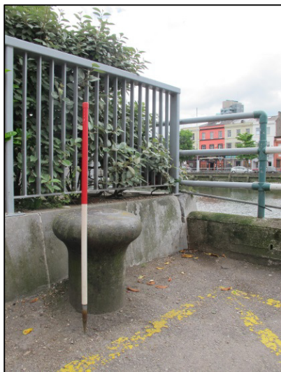
Plate 25: South-facing view of cast-iron mooring bollard located towards the southern end of Morrison's Quay (1m scale).
